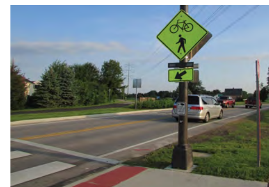
An example of a crosswalk with rectangular rapid flashing beacons Image Source: U.S. Department of Transportation
