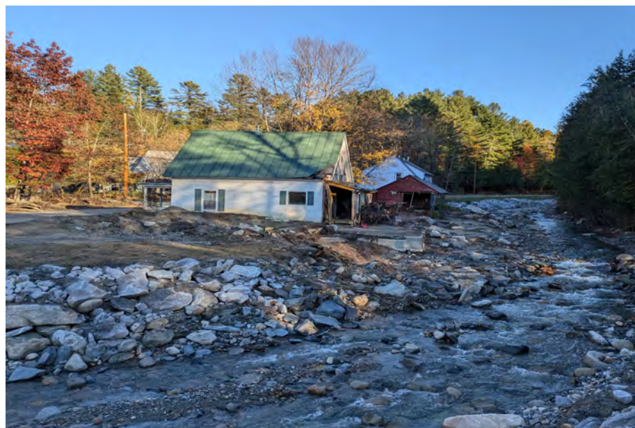
Flood Damage in Plainfield; Image Source: Plainfield Studio
